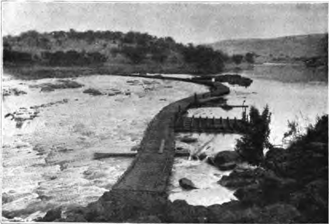
BRIDGE OF SLEEPERS TAKEN UP FROM THE MAIN LINE OF THE NATAL GOVERNMENT RAILWAYS, THROWN OVER THE TUGELA BY THE BOERS
